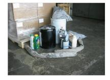
3. Non-porous surface mixing and cleaning area with no curbing (dike) or sump; spill absorbent materials are kept nearby.
