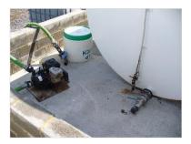
Non-porous surface mixing and cleaning area has curbing (dike) and emergency spill collection sump and pump; spill absorbent materials nearby.
