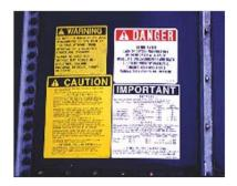
Sign is made from paper, metal, or plastic; does not contain pictogram; is prominently displayed near access point(s); is faded and hard to read.
