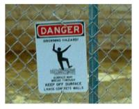
5. Sign is made from plastic or metal; includes pictogram of the hazard; is prominently displayed near access point(s); is easily read.
