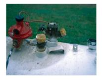
5. Valves are clean, rust free, and operate properly. Tank is protected by an earthen, metal, or wooden berm.
