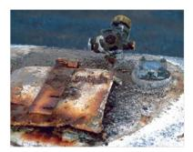
3. Valves have some debris or rust on them; valves work properly but tank is not protected by an earthen, metal, or wooden berm.
