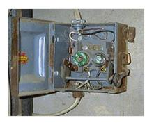
Panel uses circuit breakers or fuses; electrical panel has some dust, trash, or spider webs on it; electrical panel cover is not securely attached.
