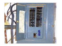
5. Panel uses circuit breakers; electrical panel is free of dust, trash, or spider webs; electrical panel cover is securely attached.
