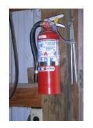
3. Only one 10-pound ABC type extinguisher is available or charged; extinguisher is not easily accessible, not mounted; only Class A or Class BC extinguishers are present.
