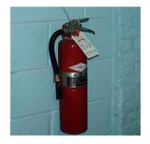
5. A 10-pound ABC type extinguisher is accessible on each floor of a building or within 50 feet of a structure; is mounted; fully charged.
