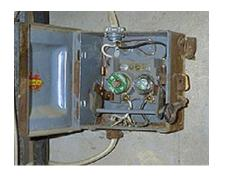
3. Panel uses fuses; electrical panel has some dust, trash, or spider webs on it; electrical panel cover is not securely attached.
