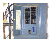
5. Panel uses circuit breakers; electrical panel is free of dust, trash, or spider webs; electrical panel cover is securely attached.
